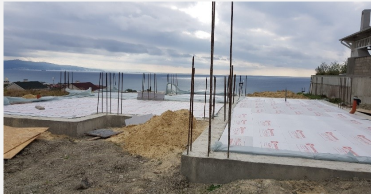
Reinforcement of the foundation of a multi-story house, Novorossiysk, 2018 Products used - composite basalt rebar with Ø10 and 14 mm
