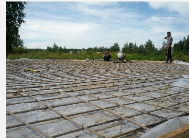
Reinforcement of the foundation of a private house, "Cottage village "Fortuna", Khabarovsk region, 2013
