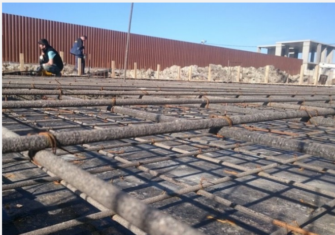
Reinforcement of the building foundation, Gelendzhik, 2017
