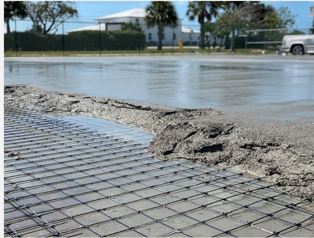
Florida Keyes Airport, Aircraft Hangar Construction
