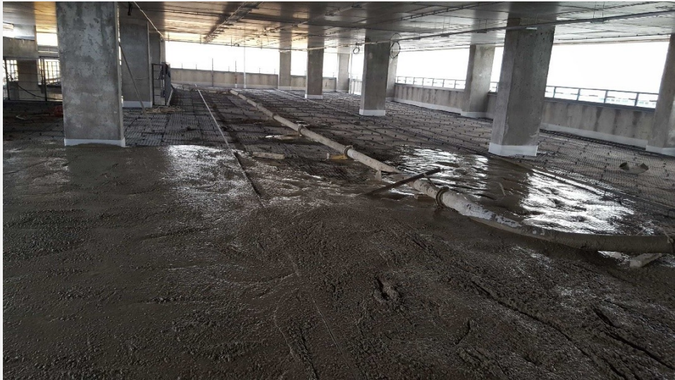
ROCKMESH® composite mesh in concrete reinforcement of a three-tier parking, Moscow, 2017
