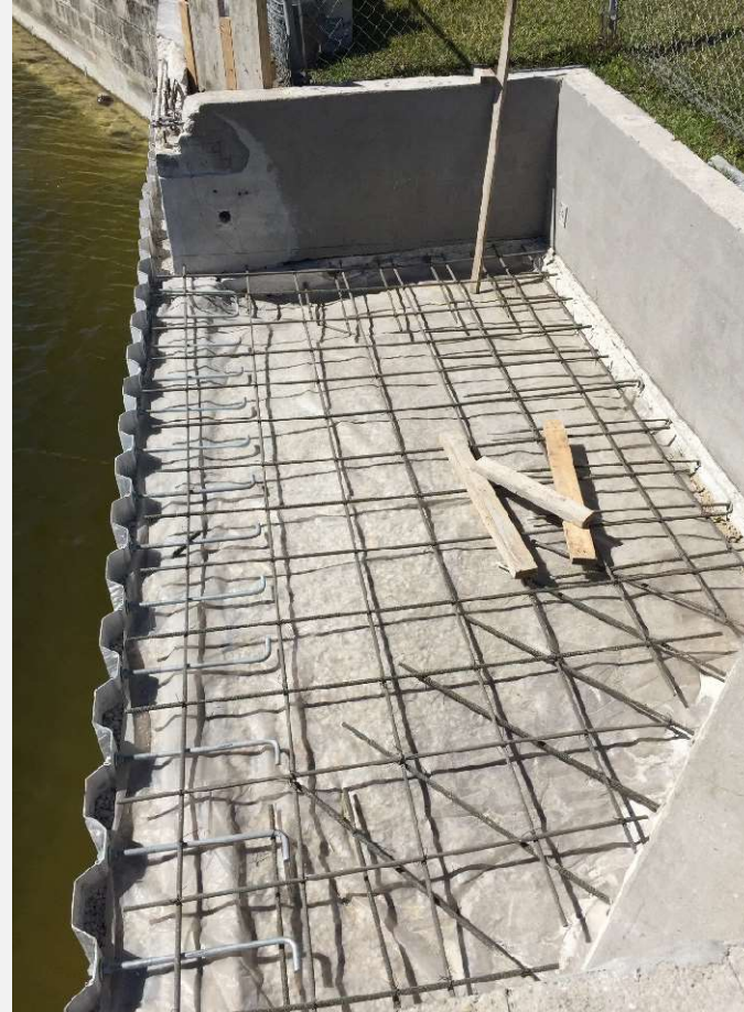
Seawall Plate reinforcement project. Composite rebar and mesh were used
