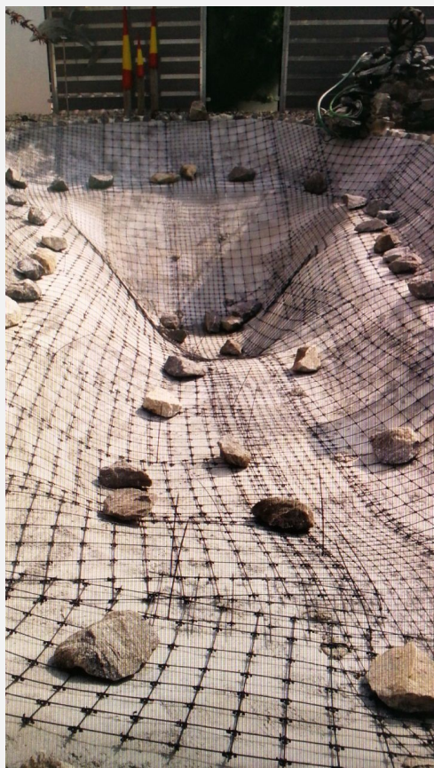
Germany, 2017 Composite mesh \varnothing 3 mm / 100x100 mm
