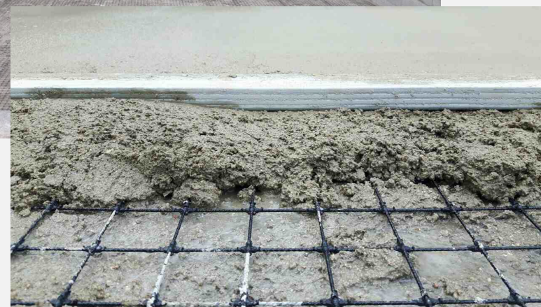
Moravská Chrastová, Czech Republic, 2017 Composite mesh \varnothing 3 mm / 100x100 mm
