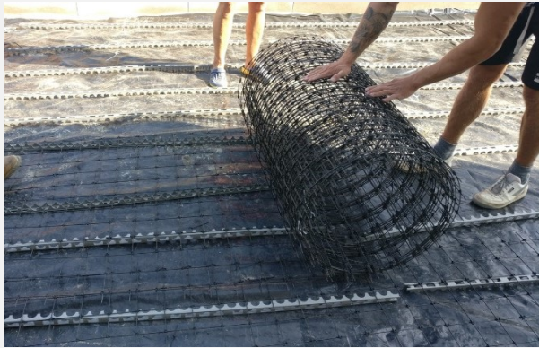
Tišnov, Czech Republic, 2018 , reinforcement of the access road with the use of composite mesh
