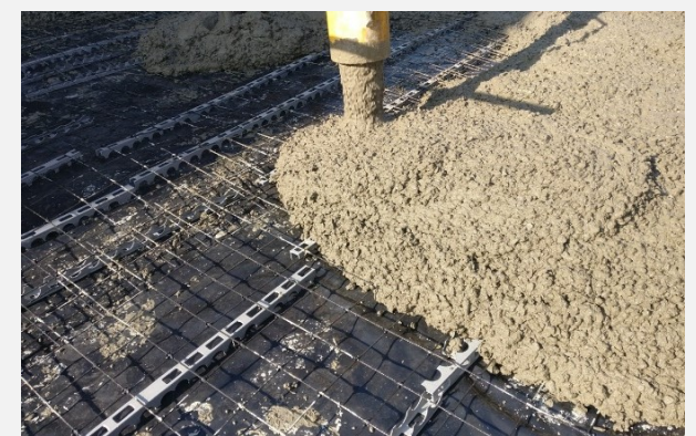
Tišnov, Czech Republic, 2018 , reinforcement of the access road with the use of composite mesh
