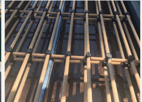
Non-standard size composite mesh with and without sand-coating
