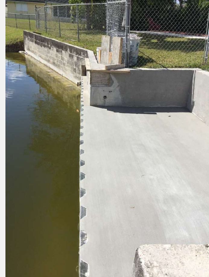
Seawall Plate reinforcement project. Composite rebar and mesh were used
