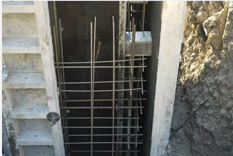
Construction of a wall of the bank stabilization structure, Russia, Novorossiysk, 2012
