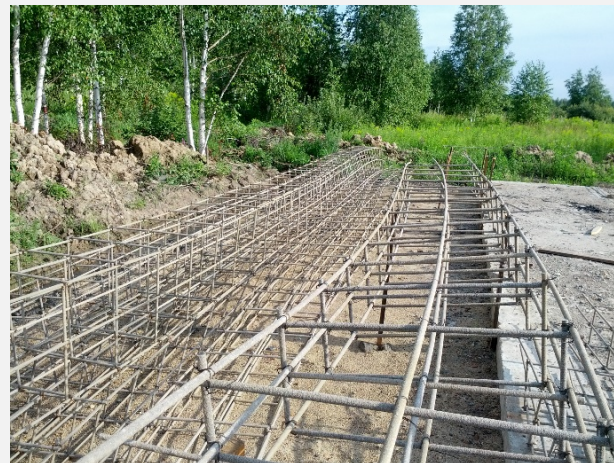
Reinforcement of the foundation of a private house, "Cottage village "Fortuna", Khabarovsk region, 2013
