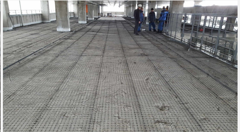
ROCKMESH® composite mesh in concrete reinforcement of a three-tier parking, Moscow, 2017
