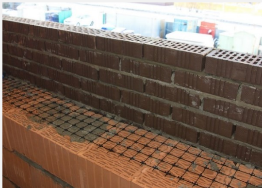
ROCKMESH® composite mesh in concrete reinforcement of a three-tier parking, Moscow, 2017
